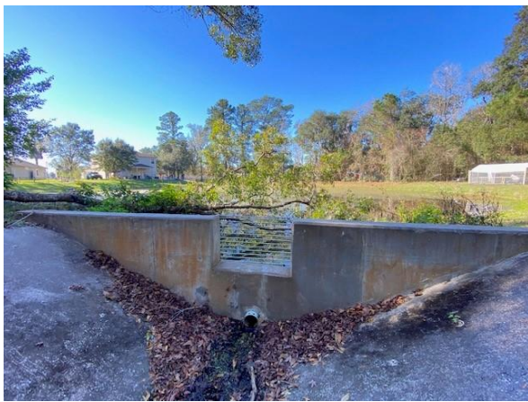
Clear debris from concrete ditch paving.
