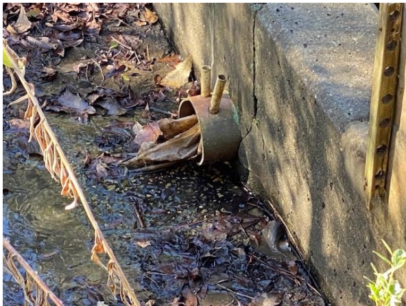
Remove debris from bleed down pipe.
