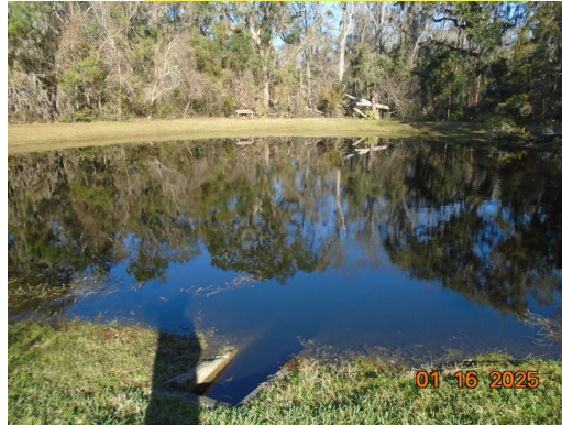
Pond 8: Outflow was clear...tree should be removed.
