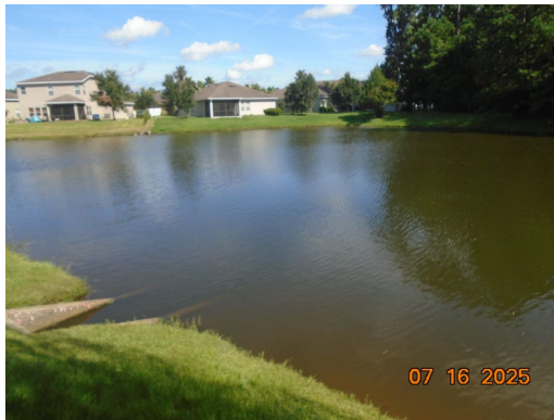
Pond 5: Pond was in good shape. Level and clarity were normal, and the outflow was in good shape.
