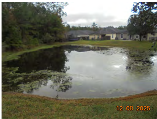
Pond 6: Pond was in good shape. Minor algal bloom to be treated once launch is dry enough.
