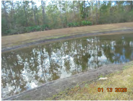
Pond 20: Pond in good condition. Level was high and clarity was normal.
