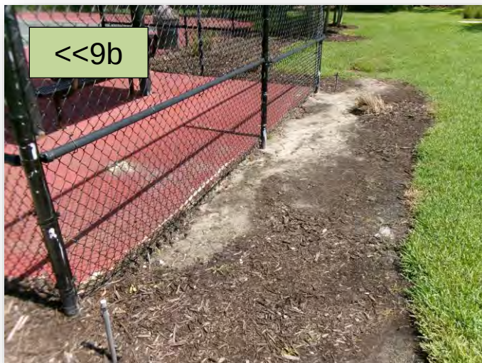
10. Crape Myrtle at the West exit of the Amenity Center should be tipped back from the roof to prevent damage.(pic.10)
